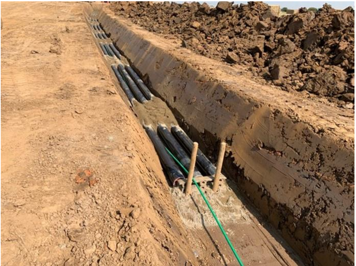
Figure 3.18: Example of an onshore export cable trench.
