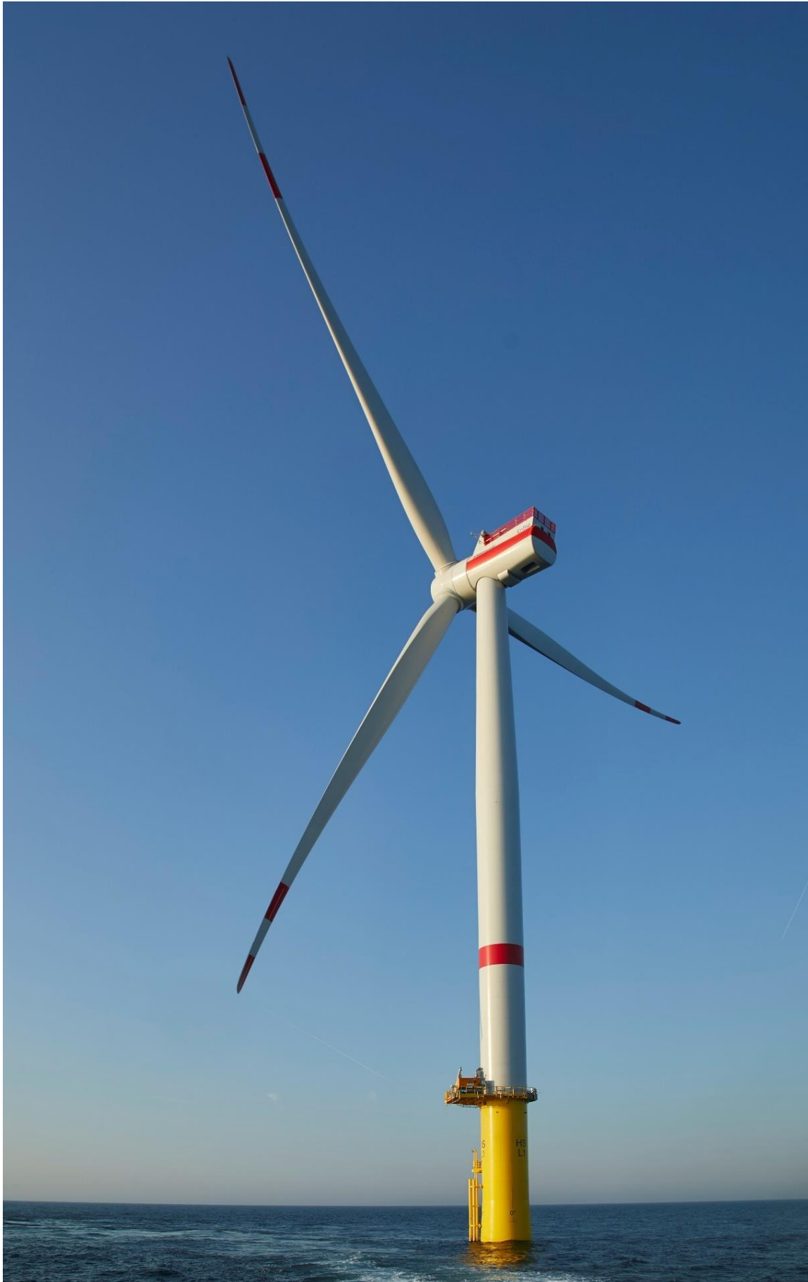
Figure 3.4: A picture of a wind turbine at the EnBW Hohe See Offshore wind farm in the German North Sea.
